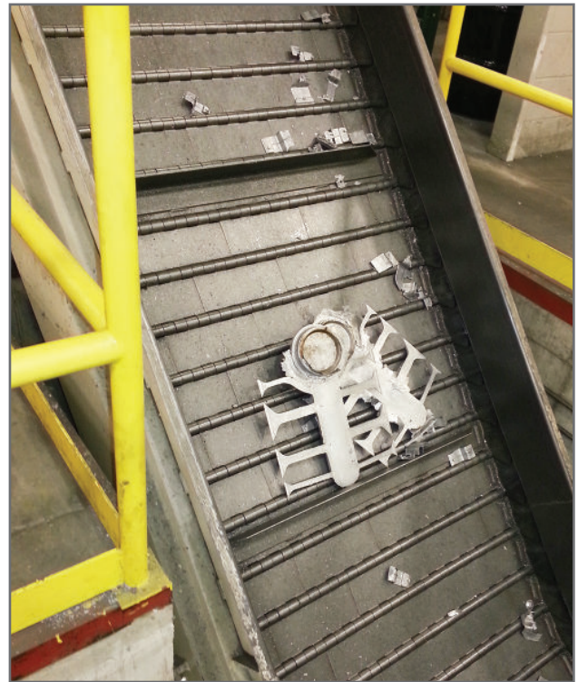
Trim scrap elevated toward the furnace on a 2 1/2" Pitch Steel Belt Z-Style Conveyor.
