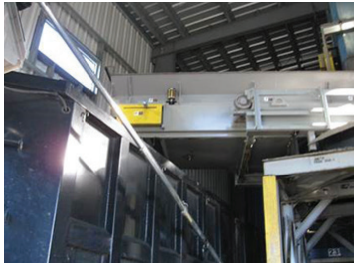
Shuttle Conveyor with extension arm and level sensors evenly fills each container.
