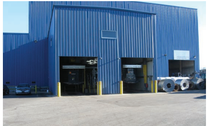
Newly completed load-out system maximized container fill and returns.
